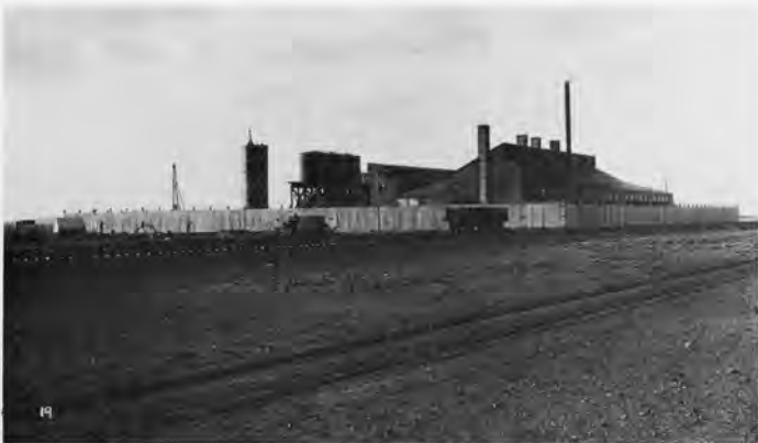
FIGURE 5—Vanadium Mines Company leach plant at Cutter, New Mexico, on the Atchison Topeka & Santa Fe Railroad. The two products of this plant, lead sulfate and vanadium pentoxide, were to be shipped to paint manufacturers and to the company's Rankin, Pennsylvania, ferro-vanadium plant, respectively. The company went to great efforts to exclude the view of curious passersby—note the high wooden fence surrounding the entire plant. Photo courtesy Mrs. Lydia Key, Black Range Museum, Hillsboro.
