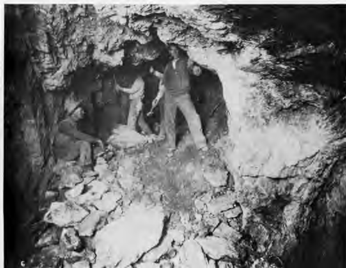
FIGURE 3—Single-jack drilling in a stope at Palomas Gap, probably in the White Swan, ca 1910. The White Swan was ultimately developed down to the 500 ft level, the Dewey to 400 ft. Photo courtesy Mrs. Lydia Key, Black Range Museum, Hillsboro.
