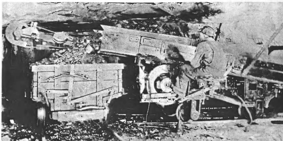
Scraper loader operations deep underground at the Stag Canyon Branch in 1929. It was an early example of new coal-mining mechanization to increase production and reduce costs.
